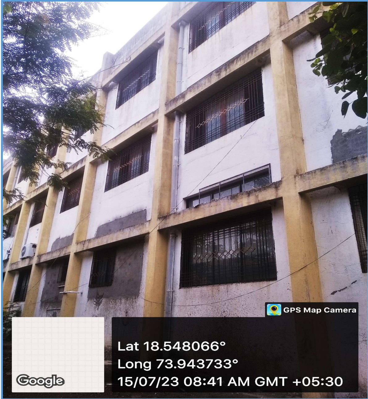
Rain Water Harvesting System
